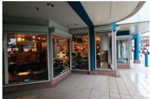
During operating hours, Talius rollshutters retract completely to provide an unobstructed view.
